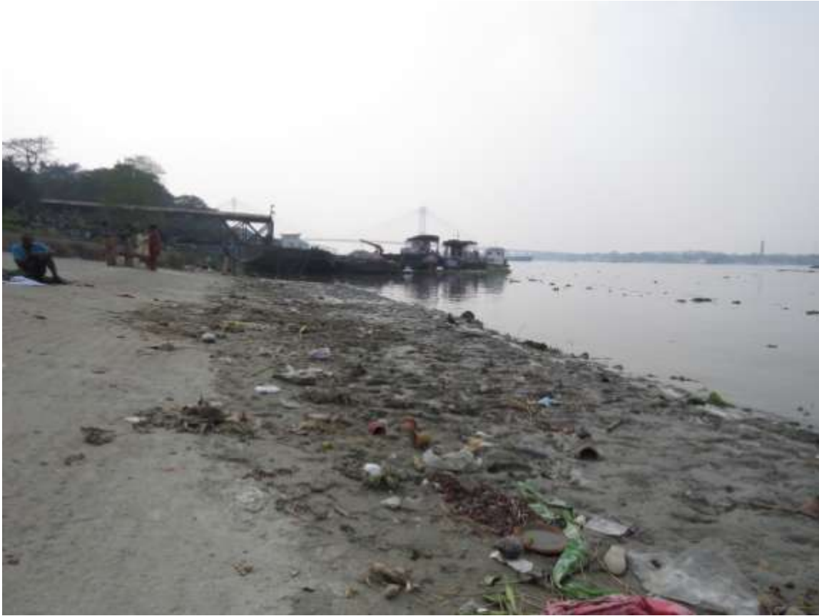
Plate 203 – Condition of Embankment near Judges Ghat
