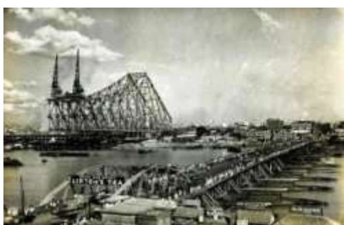
Plate 79: Construction of Bridge (Source BBJ Website)
