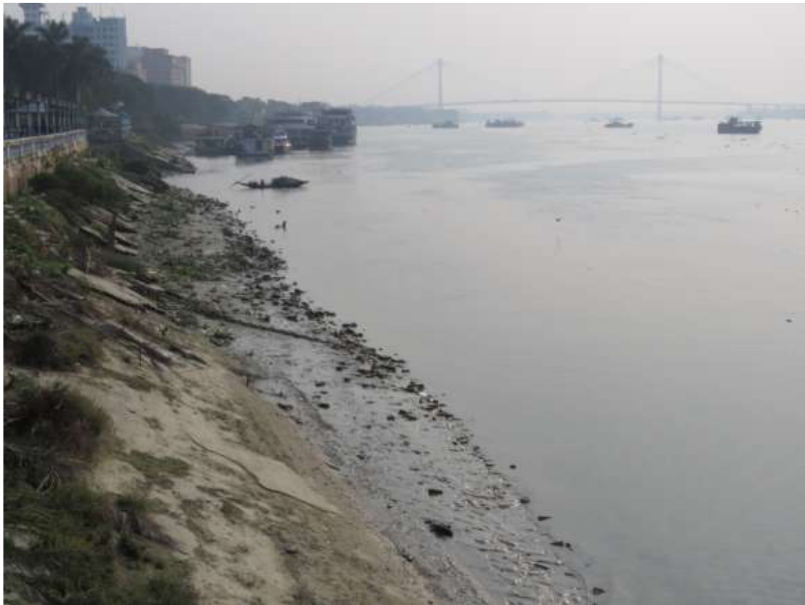
Plate 201 – Embankment near Millennium Park
