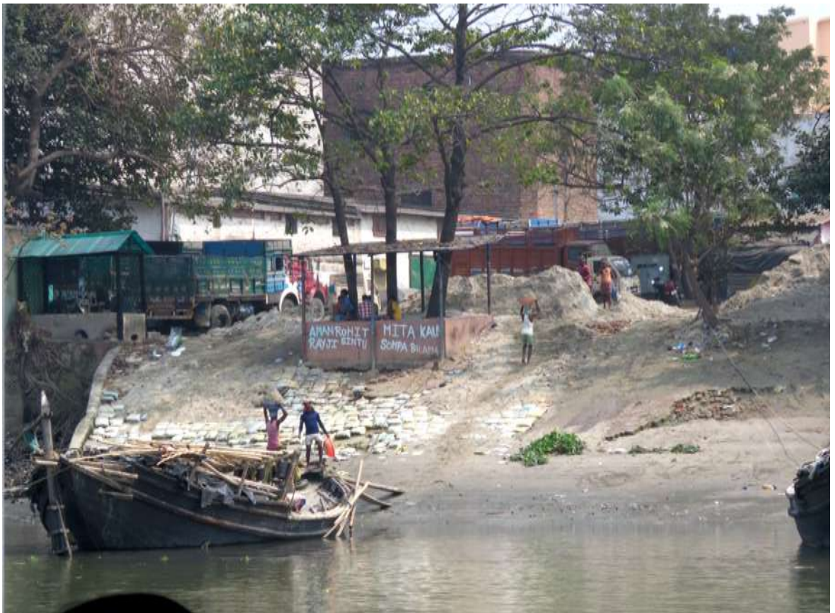
Plate 191 - Condition of Embankment in Bagbazar Ghat
