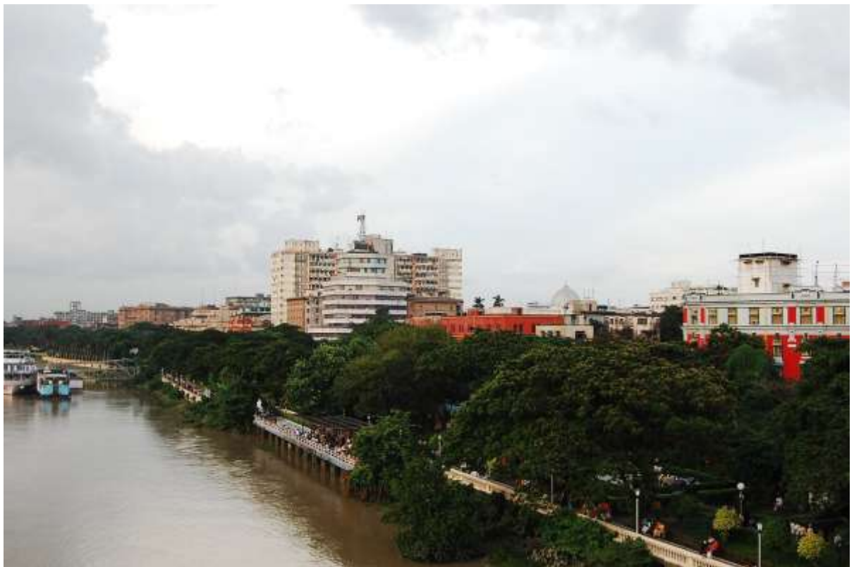
Plate 161 – Commercial Built up area, along Hugli River, Source – Kolkata Police
