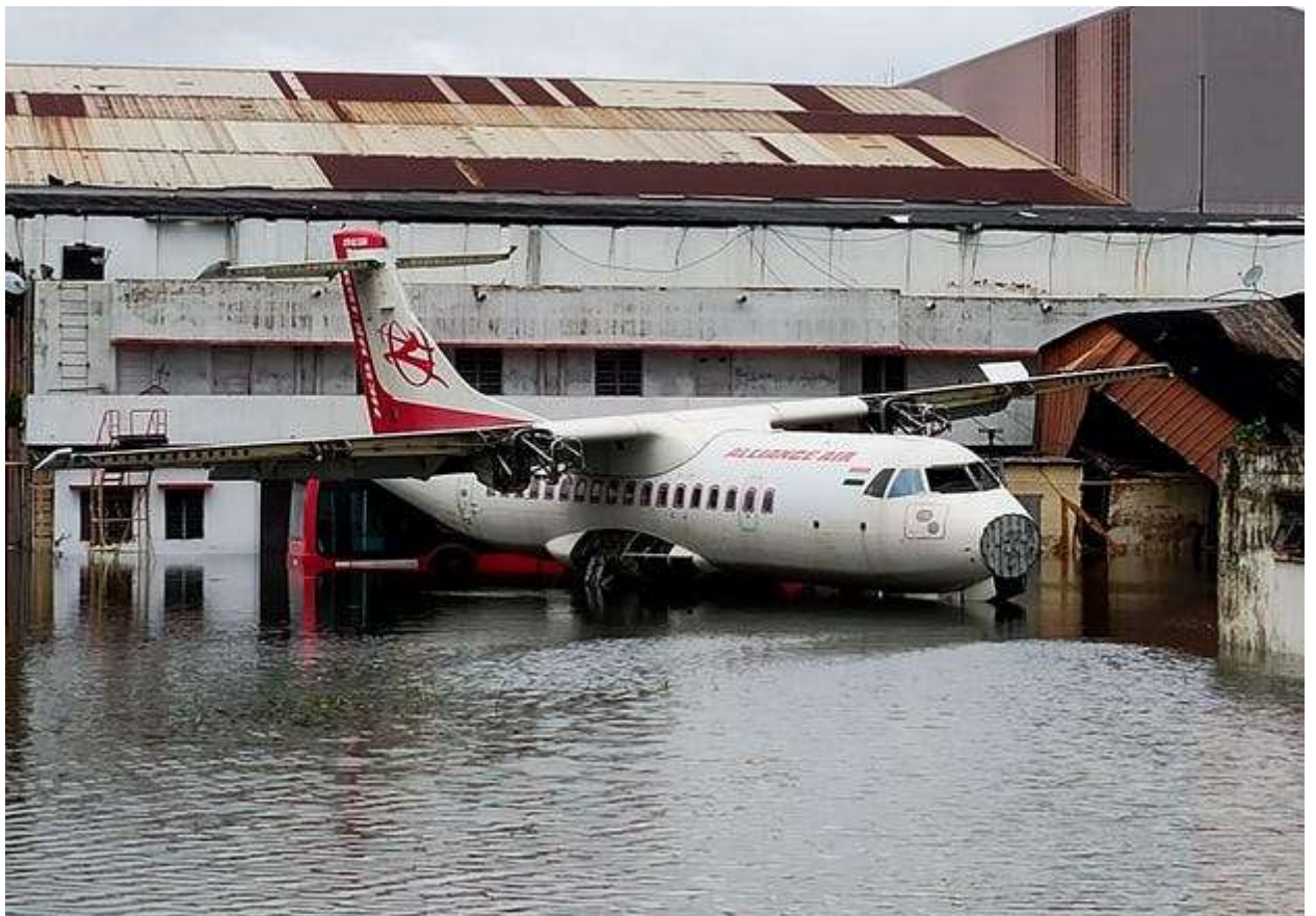
Plate 187: Flooded Airport , Dumdum
