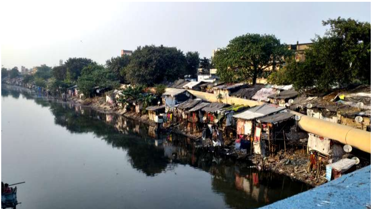
Plate 32 –Encroached Bank of Circular Canal , 22°34'57.27"N 88°23'18.55"E
