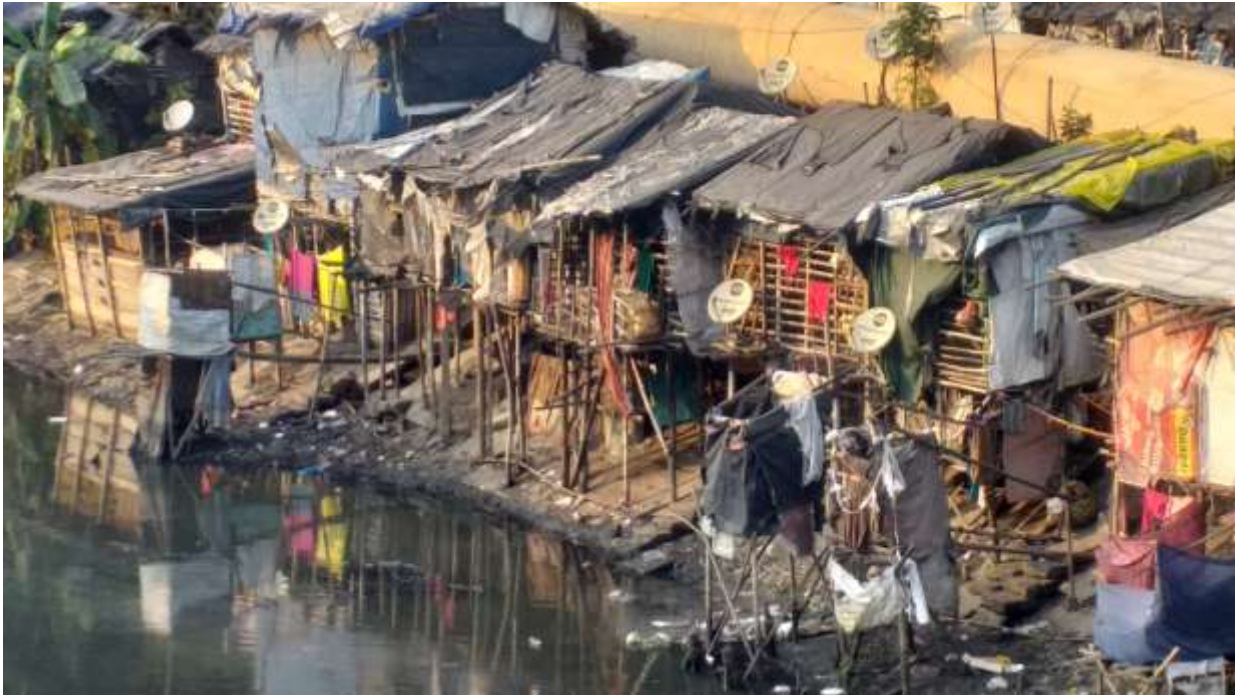
Plate 222: Encroached Canal Banks
