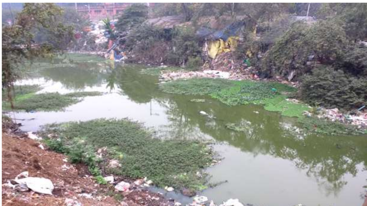
Plate 31– Condition of Beliaghata Canal, 22°34'8.05"N 88°22'45.29"E
