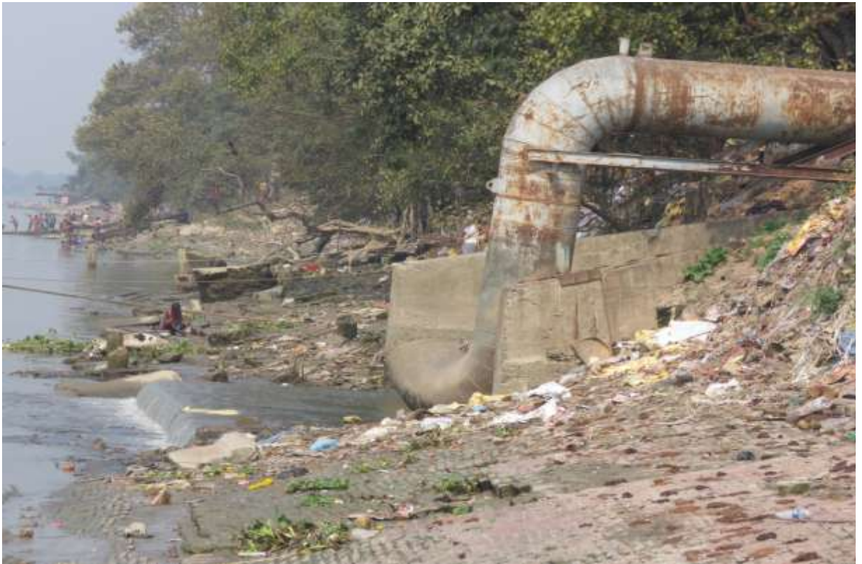
Plate 213: Sewage Outfall near Jagannath Ghat
