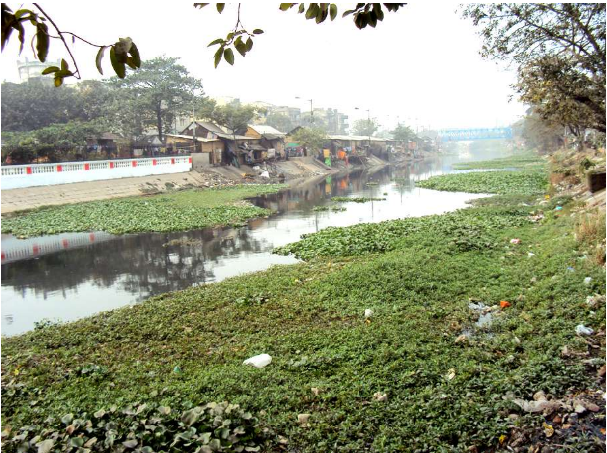
Plate 35: Present Condition of New-Cut Canal, near R.G Kar Hospital, 22°36'11.91"N 88°22'37.07"E
