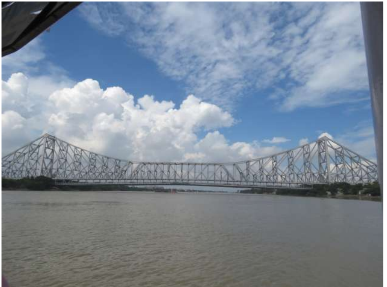
Plate 5 – The present view of Hugli River with the Iconic Howrah Bridge
