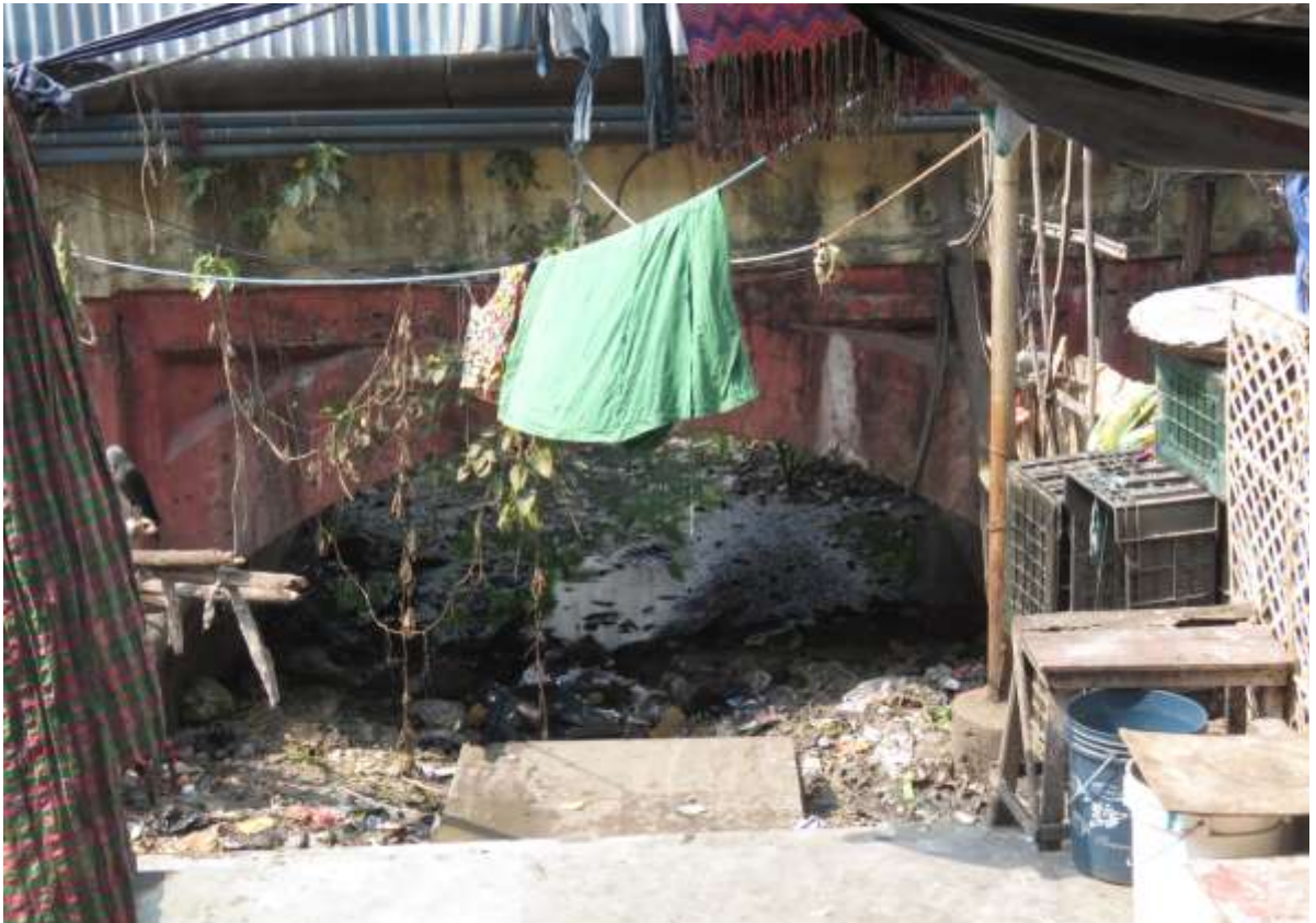
Plate 215: Sewage Outfall near Babughat
