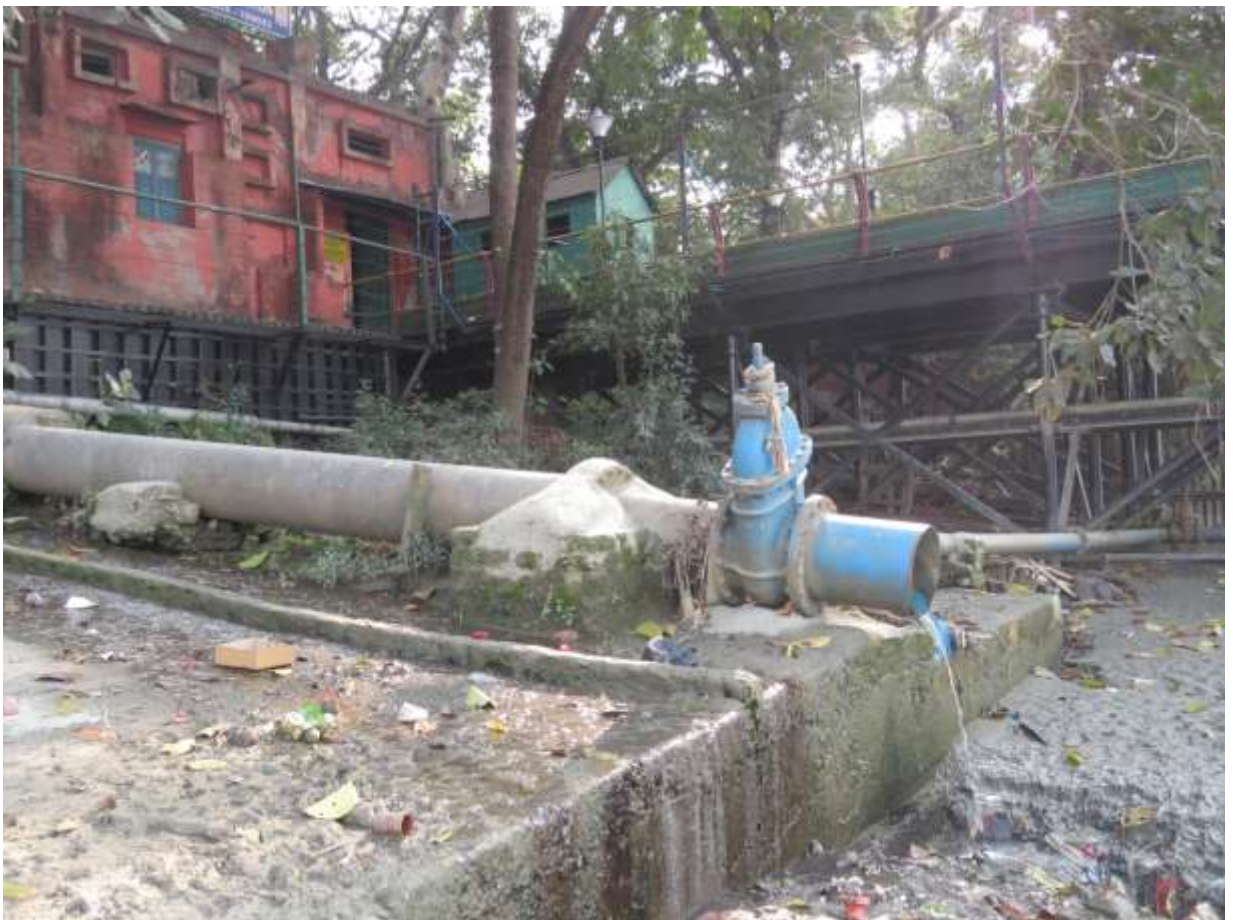
Plate 216: Sewage Outfall near Watganj
