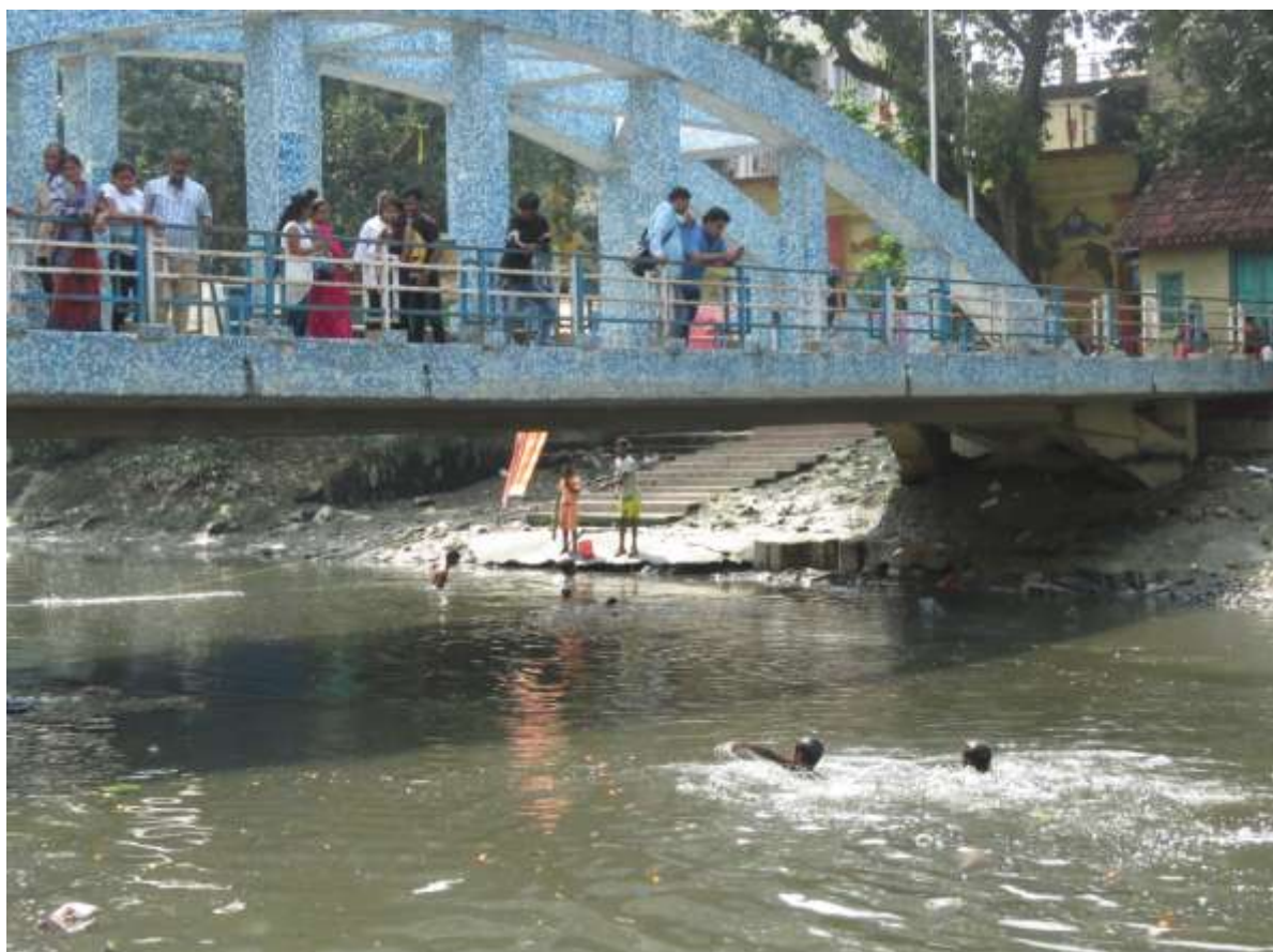
Plate 92 – The New Bridge on Adi Ganga replacing the old Boat Bridge, Kalighat
