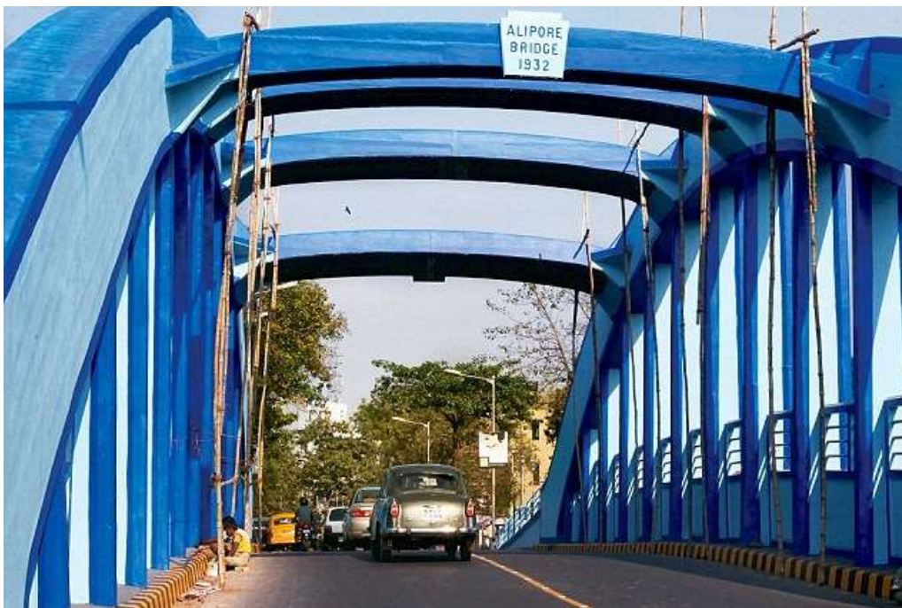
Plate 89: Bridge on Adi Ganga near Dai Ghat, Plate 90 –New Alipur Bridge, 1932
