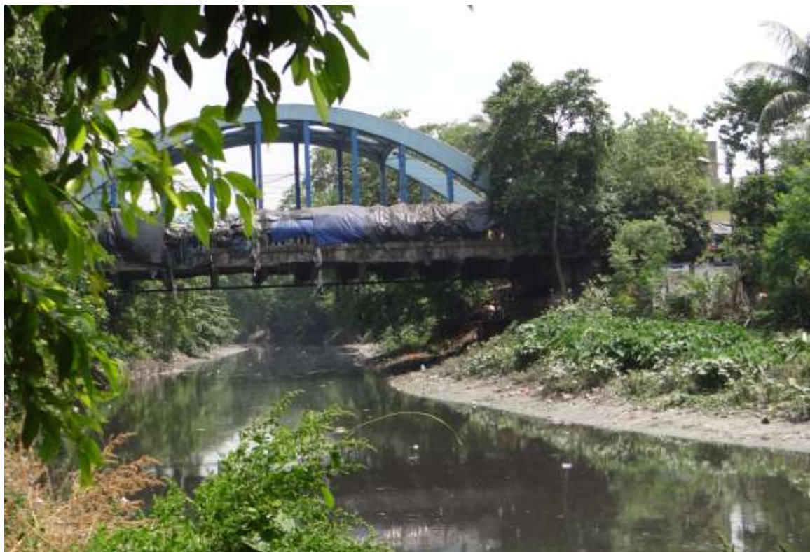
Plate 48: Near Baro Ras Bari Ghat along Adi Ganga, Chetla 22°30'39.03"N 88°20'24.79"E
