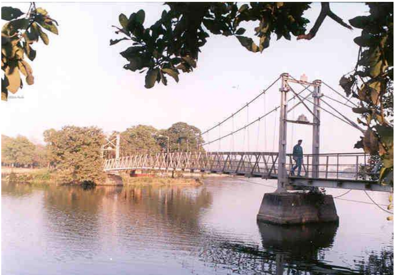
Plate 95 – A cable-stayed bridge, constructed by Burn & Co. in 1926, at the Rabindra Sarobar Lake, Kolkata (Website – BBJ)
